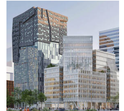
The CubeHouse , delivered 2025 Hybrid timber office Amsterdam
